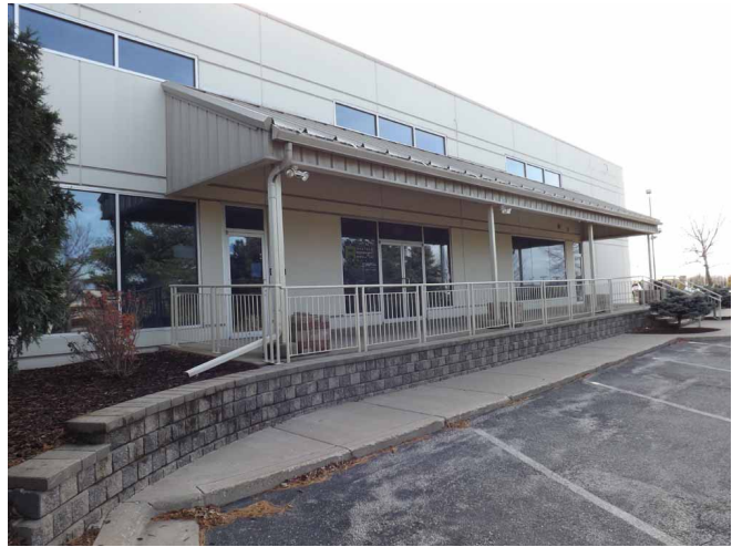
Building north elevation
