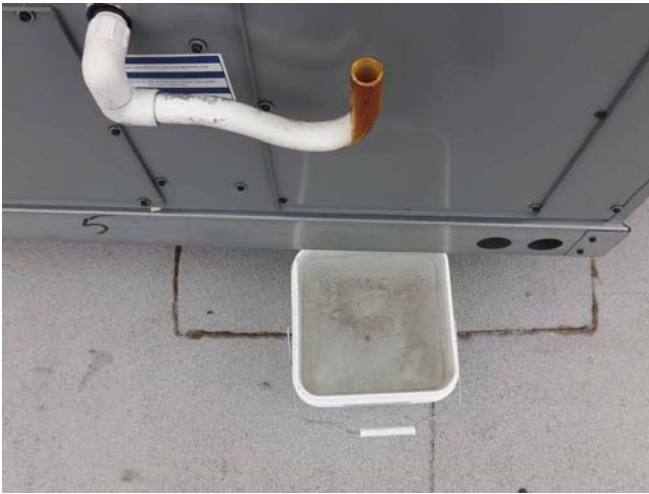
Bucket w/ice water from condensate drain line above
