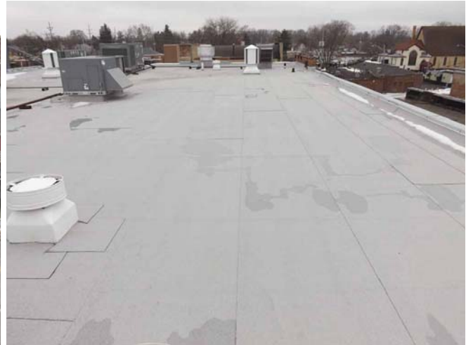
Field of MB roof above the restaurant
