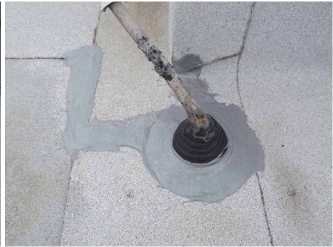
Sealant applied to lap joints and roof penetration
